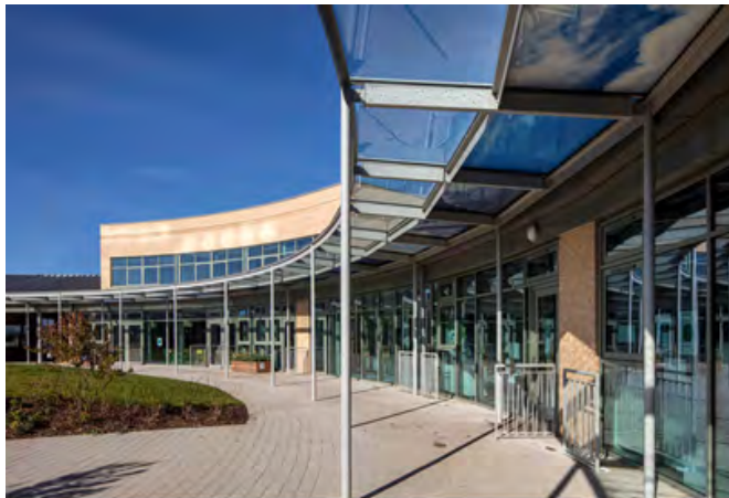
Shading device at University of Cambridge Primary School. Source: University of Cambridge, Eddington, Cambridge
