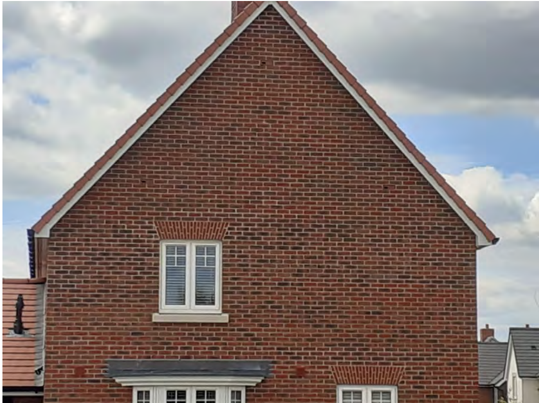
Bat and bird bricks on the gable end of new houses in Buckinghamshire Source: Herts and Middlesex Wildlife Trust
